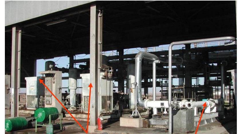
Installed SJP after compressor removal
